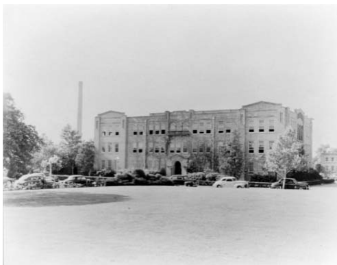
Ransom Hall at UTA, built 1915
