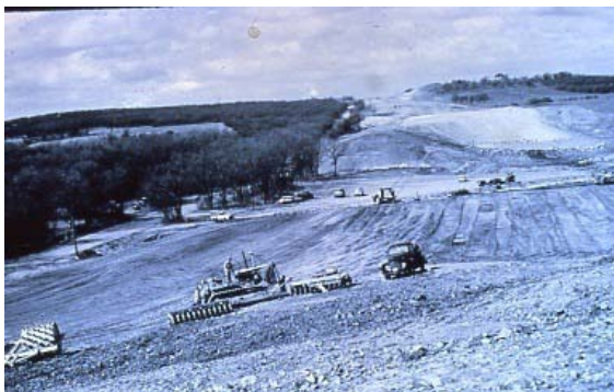
Dallas-Ft. Worth Turnpike under construction, ca. 1956
