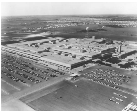
General Motors Plant, looking southwest
