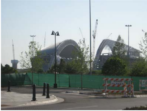
Cowboys football stadium under construction Spring 2008
