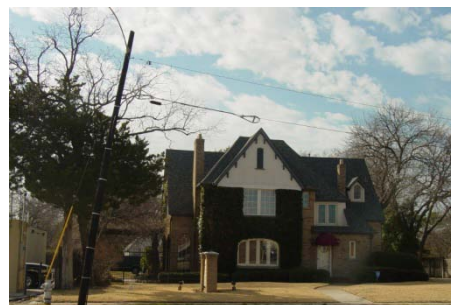
Old Mayor's House on East Abram is one of several restored by Xavier Carrillo.
